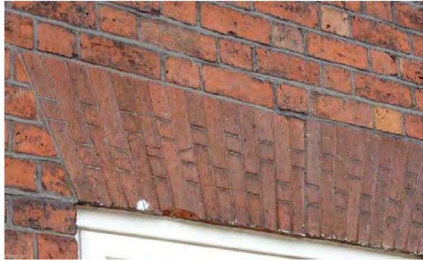
In the 18th century, where wealth permitted in the finer houses, “hand-rubbed” bricks or “gauged” bricks were used. The result was a precise, thinly-jointed, wedge-shaped lintel. Originally, the brickwork joints (including false joints) were picked out in a fine white lime mortar or “putty”, which in most cases has weathered away (left and above). The example at 50 High Street (below) is an early 20th century copy.
