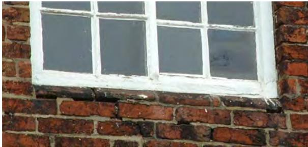
Above - where there was no cill, as with many of the smaller cottages and the less important elevations of the town houses, the window joinery was positioned close to the face of the wall. In the example above handmade bricks were moulded to create a weathering.
