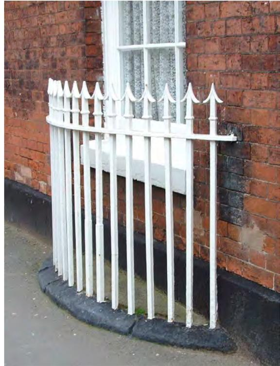
Although most of the railings have been removed, many gates were retained and these incorporate cast-iron posts with ball tops and urns and railings with hoops, spear-tops, buds and spikes. These provide detailed evidence of the former appearance of the railings.
