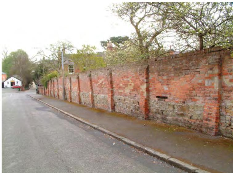
Most of the boundary walls serving domestic properties within Repton are built from red brick, with a sparing use of headers to form the bonding pattern. The example on the right is a late 19th century wall to The Priory, using English Garden Wall bond brickwork and red clay copings on an earlier wall.
