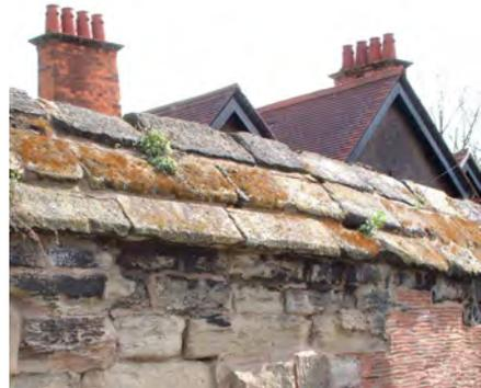
The earliest walls within the village are built from local stone, the best examples being the large blocks of stone used for the Priory precinct walls, which have wedge-shaped stone copings (right), but there are instances where rubble sandstone survives, usually on the side passages, sometimes freestanding & sometimes used for the footings of a later 18<sup>th</sup> or 19<sup>th</sup> century wall (right).
