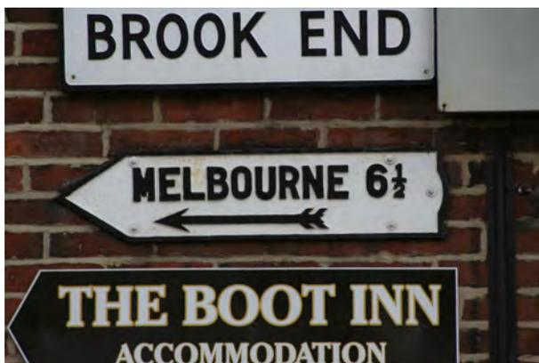
Above and bottom right - Arrow-shaped cast iron directional sign, with raised letters, arrow and mileage.
