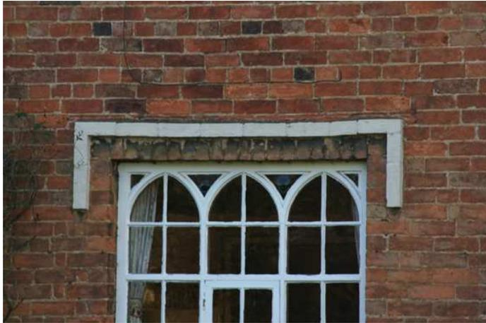
Left - hood mould constructed from painted bricks, over soldier course of brickwork forming a lintel. This window relied on the strength of the timber window to support the brickwork above.
