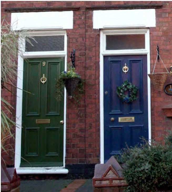
Along Main Street, during the 19th century, most of the new detached & terraced houses were built with panelled doors. Those at 9 and 11 Clifton Road (left) have four panels with heavily modelled, applied, bolection mouldings, and a plain fanlight.
