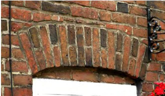
In association with casement windows, the most common pattern of lintel is the segmental brick arch. This was often used for economy. The example at The Almshouses (left) incorporates header and stretcher bricks, many of the headers have been fired at a higher temperature and so appear almost blue. The brick infill between the arch and the window, set back, is a typical early detail.
