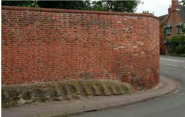
Above - The old wall on the corner of Church Street and Main Street was built on top of the bedrock. The wall at the entrance to Newlands House (right) was part built in rubble sandstone. In both cases moulded red brick copings were used. They were ideally suited to following the undulating wall head (detail below).
