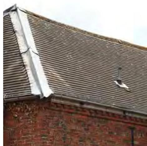
Bottom left & right - hipped tiled roofs at Netherseal Old Hall and The Stable Yard. These hips have rolled lead flashings.
