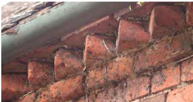
**Eaves details** - sawtooth and dentilled corbelled brickwork at the eaves are common details. Left - sawtooth brickwork (The Old Hall). Left above - dentilled brickwork at The Old Stableyard.
