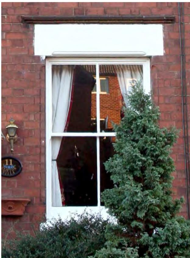
Left - 11 Clifton Road. The moulded details in the stone lintel are replicated in the terracotta window jambs.
