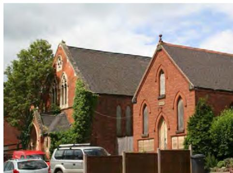
built in a Gothic Revival style of architecture, using English bond brickwork, the former using stone for the decorated windows and trefoil panels and the latter using simplified lancet windows made with moulded bricks. There is a series of engraved foundation stones in the front gable.
