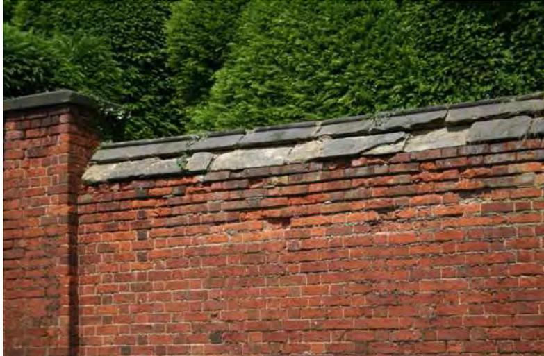
Below right - detail of chamfered, moulded stone coping at The Old Stableyard
