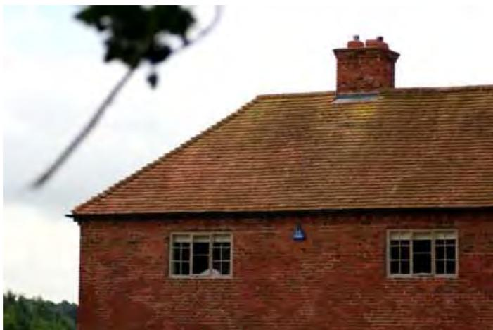
Left - hipped roof in plain clay tiles at Mill Farm, with hips of bonnet tiles.
