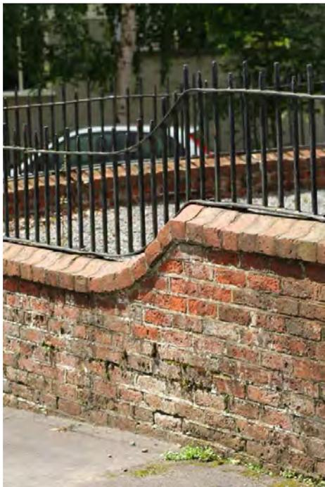
Above - estate railings of wrought iron with round bar top rail and flat bar lower rails (Church St). This type of five-bar estate railing is found in a number of places, but mainly between the private grounds & fields around the former Netherseal Hall
