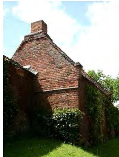
*Stepped brick parapet to roof at Grade II listed former Smithy at the Old Stableyard*
