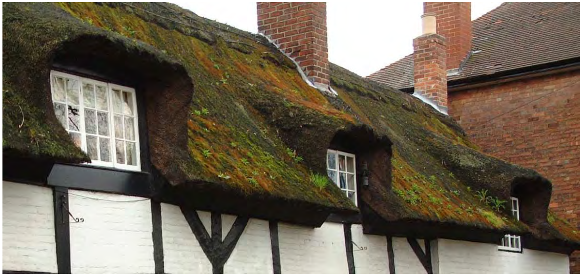
(Above) Thatched roof at 5 Willington Road.
