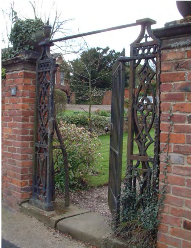
The cast-iron gateway at The Grange on Main Street (left) illustrates the early use of cast-iron at the turn of the 19th century.
