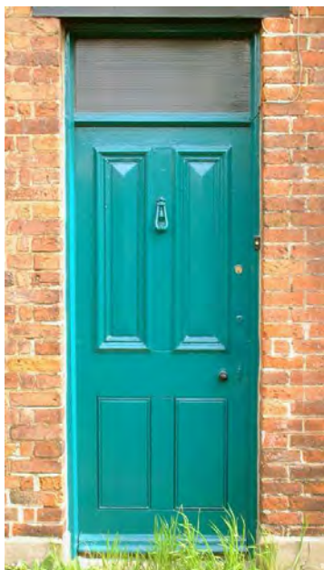
Below - 19th century Victorian panelled doors. From left; (1) Four-panel with bead mouldings to bottom panels and raised panels above, with “bolection” mouldings, (2) Panelled former shop door with bead mouldings. The glazed panel has been boarded over. (3) Three-panel with heavy “bolection” mouldings.
