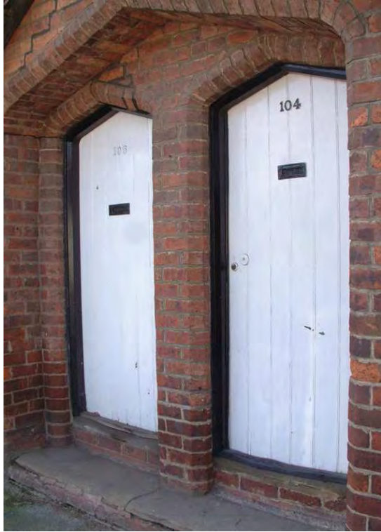
Above left - pair of fully boarded 19th century doors, a style appropriate for Gothic style cottages (104-106 High Street). Above right - pair of 19th century boarded and framed doors with applied fillets (94-96 High Street). This style was also adopted for its Gothic characteristics.
