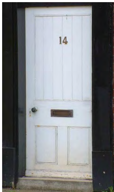
Below - 19th century Victorian panelled doors. From left; (1) Four-panel with bead mouldings to bottom panels and raised panels above, with “bolection” mouldings, (2) Panelled former shop door with bead mouldings. The glazed panel has been boarded over. (3) Three-panel with heavy “bolection” mouldings.
