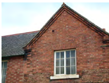
Left - pitched roof with corbelled brick verge
