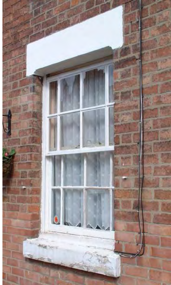
Above - late 19th century squared stone lintel with chamfered bottom edge and stone cill. By this date the sash box frame was set back behind the brick reveal.
