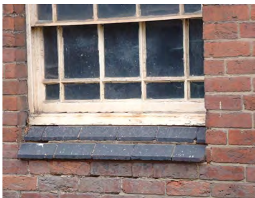
In some cases, moulded blue bricks were added to form a more weatherproof cill. The example shown below dates from the second half of the 19 th century and the cill is part of the original construction.
