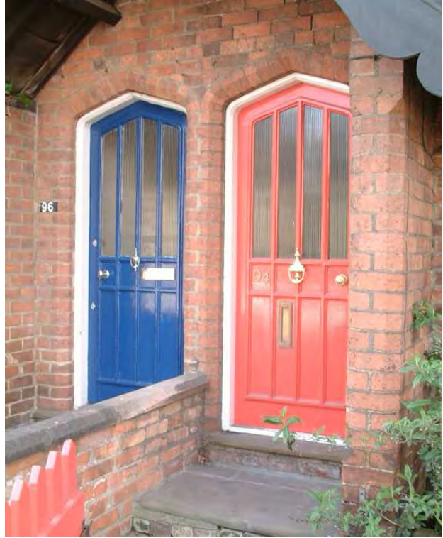
Above left - pair of fully boarded 19th century doors, a style appropriate for Gothic style cottages (104-106 High Street). Above right - pair of 19th century boarded and framed doors with applied fillets (94-96 High Street). This style was also adopted for its Gothic characteristics.
