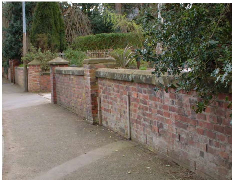
Brick wall and stone coping at Holly Bank, Main Street (below)
