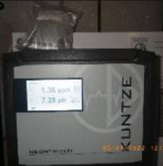
A photograph of a KUNTZE pH meter. The digital display shows a pH reading of 7.28. The meter is labeled "KUNTZE" and "NEON MULTI". The timestamp at the bottom right of the image reads "05/01/2022 12:29".                                   | <p>pH reading for the pool at Etwell.</p> |
