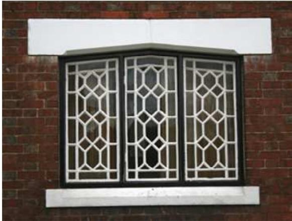
Above - side-hinged casement windows of 1864, manufactured in cast iron, at the Old Post Office, 17 Twyford Road. The complex pattern of glazing, incorporating lozenges and rectangular margin lights, is characteristic of Victorian Jacobean architecture. Cast-iron was an ideal material for this as the glazing bars were thin, enabling intricate, fine details. The shaped stone lintel, with a four-centred arched soffit, and the chamfered cill are also contemporary.
