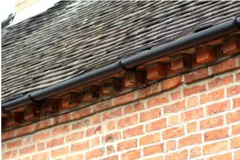
Left - dentilled brick eaves. Each alternate header brick projects to create a decorative effect.
