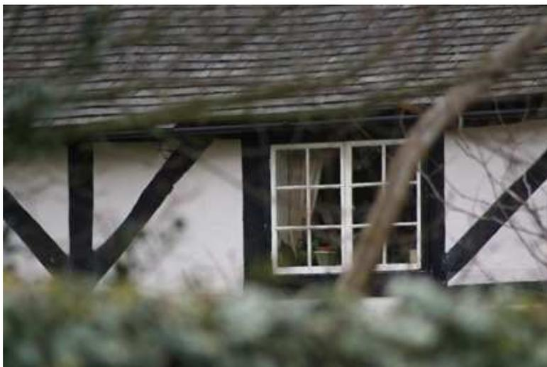
The type of frame used in this area is known as small box framing. Squared panels are made up of short lengths of horizontal rails and timber posts, jointed together. The upper storey is often braced, as in this example at St Wilfrid's, 16 Church Lane (left).
