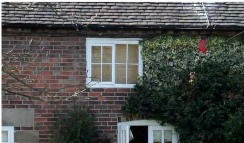
**Segmental brick arches** were commonly adopted in the 18th and early 19th centuries. This example at Trent House, Church Lane (left), incorporates incised stretcher bricks; each alternate brick is incised with a scratched horizontal line to receive a narrow “joint” of lime putty. The putty would have been added later to create the effect of an arch made of stretcher and header bricks. Modern re-pointing has removed some of the original subtlety.
