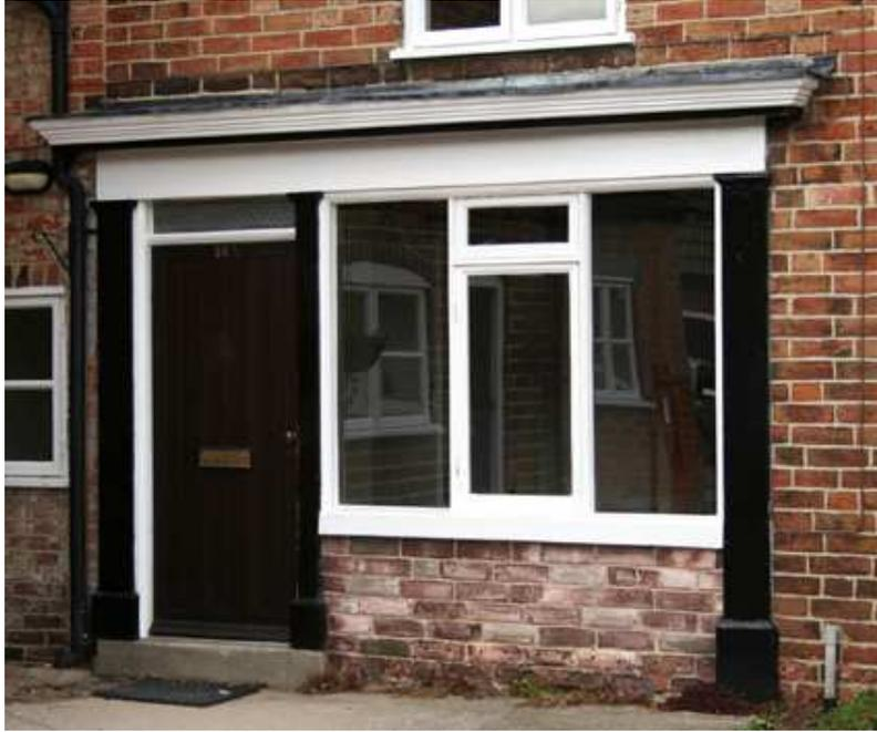
Traditional shopfront at 16 Twyford Road (left). The elements of a traditional shopfront include paired pilasters, a moulded cornice, narrow fascia and a stall-riser, which in this case is brick. The door and fanlight are original but the window is a modern replacement.
