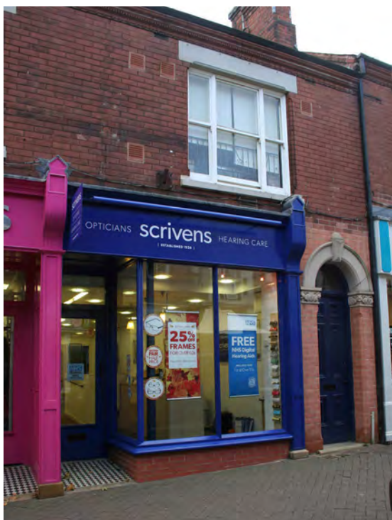
Restoration of the Edwardian shopfront at 18 High Street (right - 2014 and far right - 2005) also involved extensive works to remodel the entrance doorway to the flats and restore the arched stone decorative doorcase. As planning permission is not needed for painting, this could easily be disfigured by painting.
