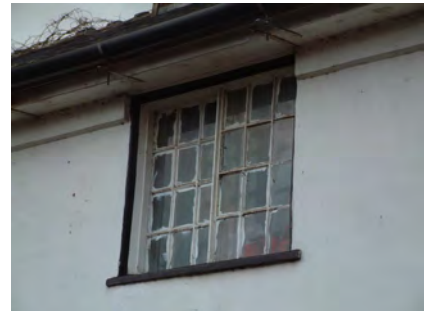
Above - horizontally-sliding multi-paned Yorkshire sash
