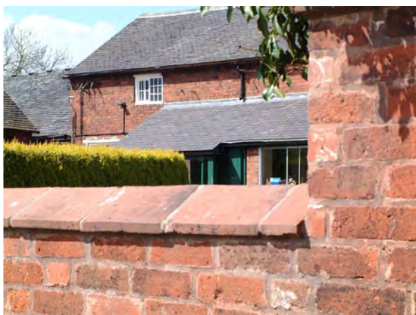
Boundary wall at Common Farm
