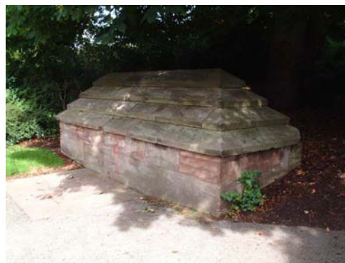
Well-head near the Church
