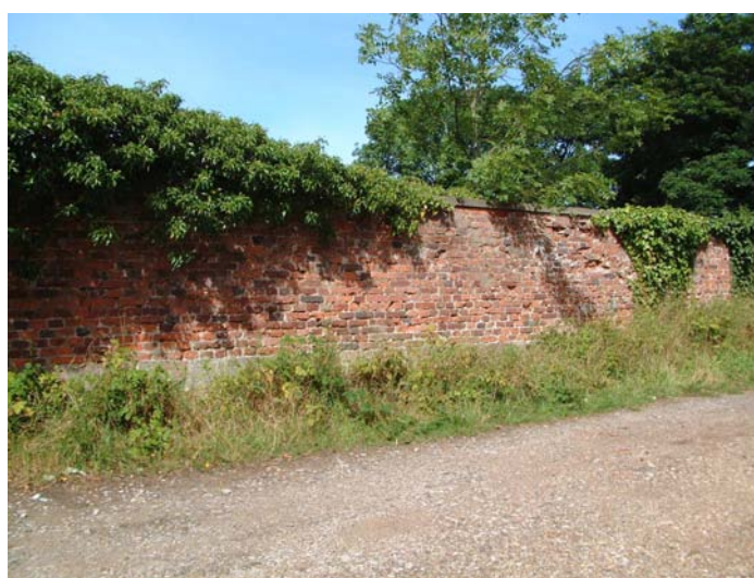
Etwall Hall - late 17th century garden wall
