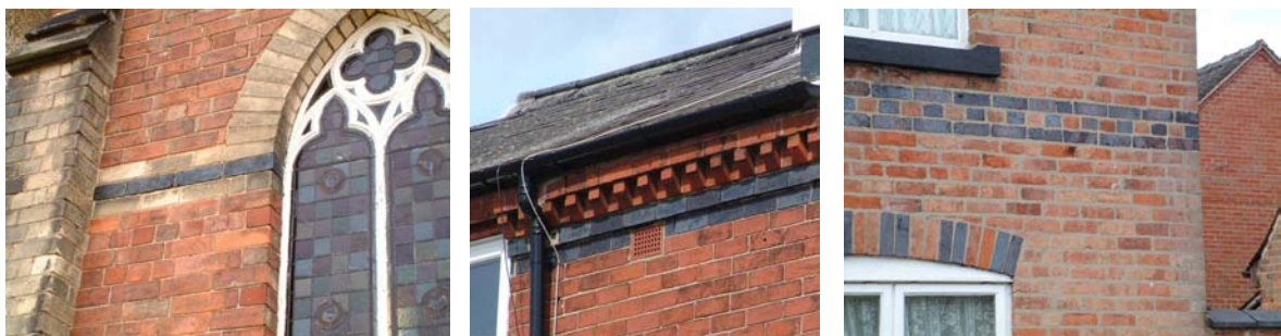
Below - small elements of buff & blue polychromatic brickwork introduced in the late 19th century.
