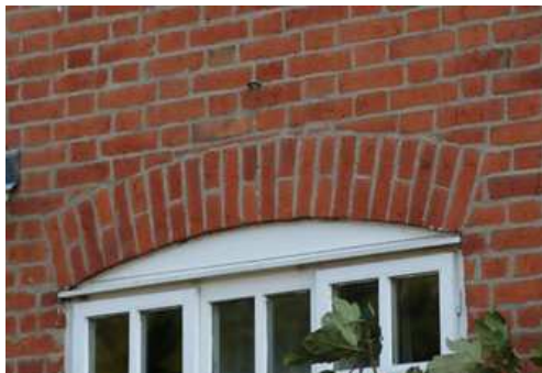
Above - segmental brick arch
