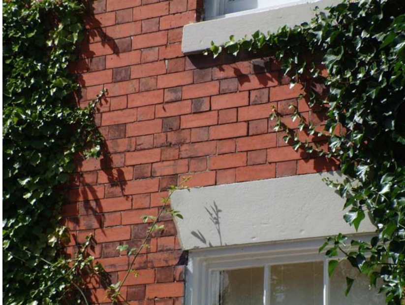
Above - mid 19th century Flemish bond brickwork.
