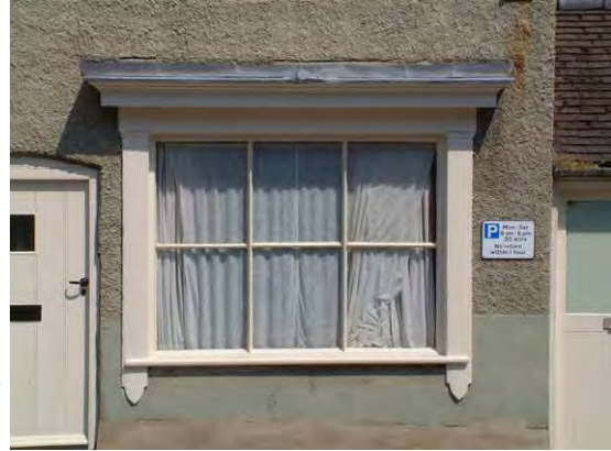
Right and above - 10 Market Place and 20 Potter Street - small "side street" shopfronts of the mid 19th century incorporating similar details; narrow pilasters, truncated at the base, a simple cornice and frieze rail and windows with glazing bars. The example at 20 Potter Street still retains its giant sash window.
