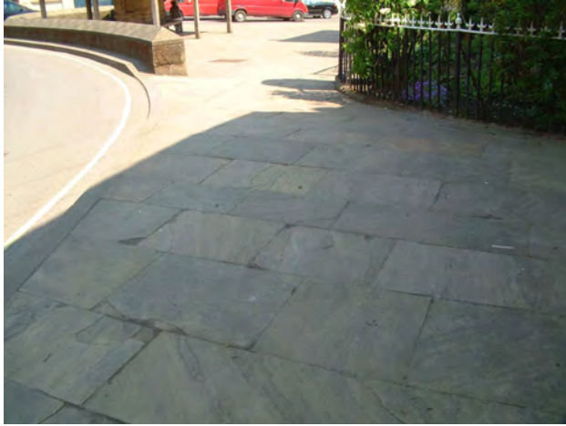
Left: Paving flags - Yorkshire (modern 20th Century riven flags from the Macclesfield area)
