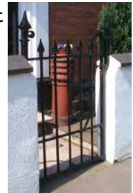
Below left - hand-forged railings in steel, fabricated in modern times to replicate the original wrought iron spear-headed pattern (15 Potter Street).
