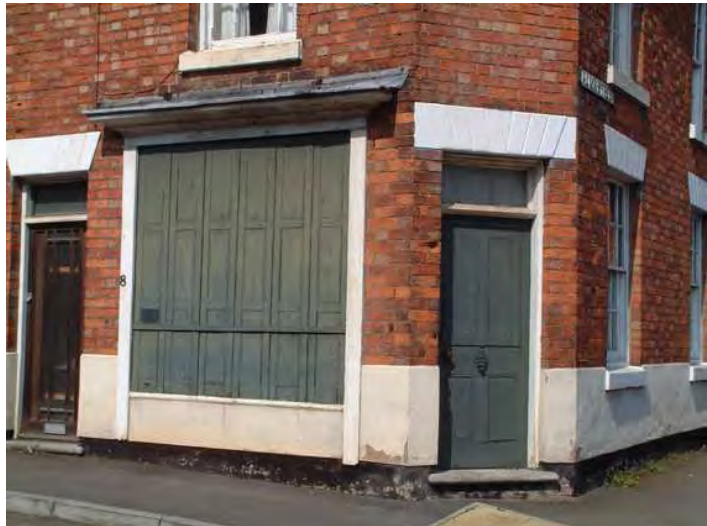
Above - a classic corner shop straddling South Street & Alma Street - the shop is now redundant but retains its historic shutters. Even the front door has its own separate shutter.
