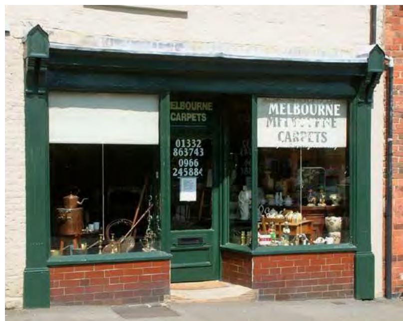
Right - Victorian shopfront at 38 High Street with brown glazed brick stall riser, decorative fluted pilasters with raised console brackets, recessed shop doorway, cornice and fascia.
