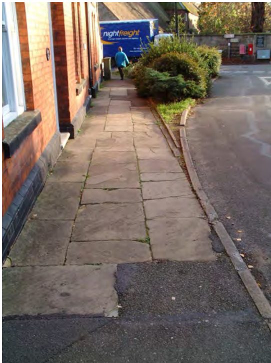
Left: Yorkshire riven paving
