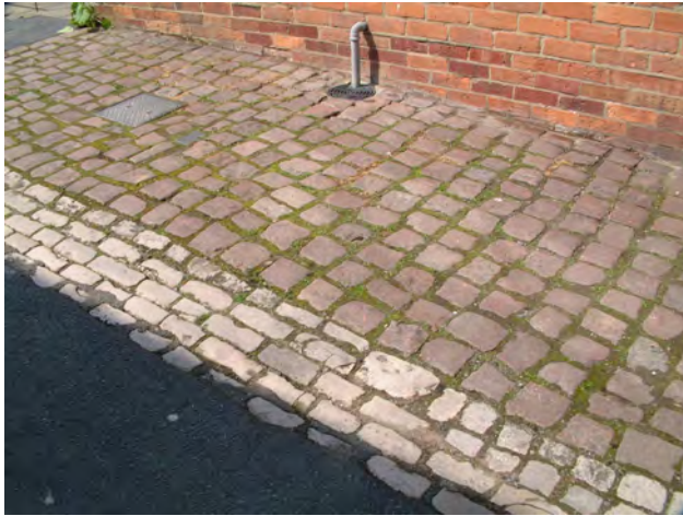
Left : Limestone sett gully
