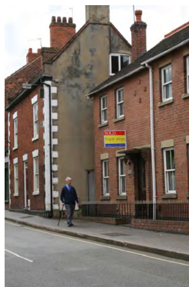
Alterations to building line
