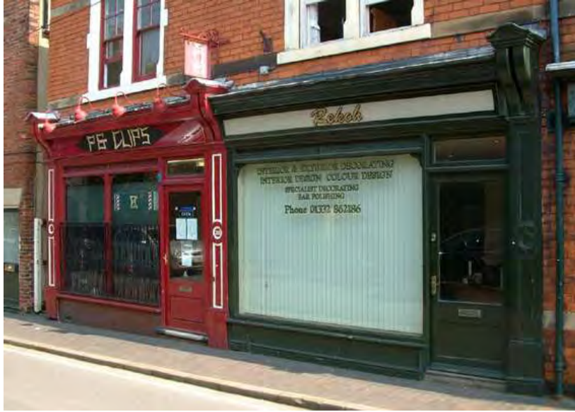
Left - Edwardian pair of identical shopfronts at 8-10 Derby Road. Heavily-moulded panelled pilasters, a bold cornice with console brackets and shop doors with fanlights. The shopfronts retain the original ventilation grilles and timber spandrels, but No. 8 has lost its central glazing mullion.
