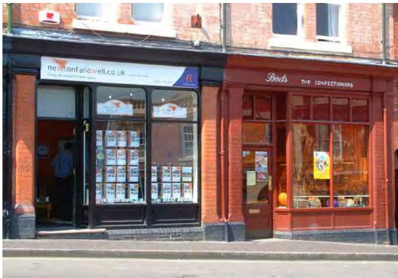
Left - Victorian shopfronts at 31-32 Market Place, originally designed as two of three matching shopfronts. The pilasters were made from moulded red bricks. The fascia and cornice was designed as one continuous run.
