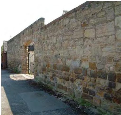
Below left - tall random rubble walls of local gritstone behind 84 High Street
