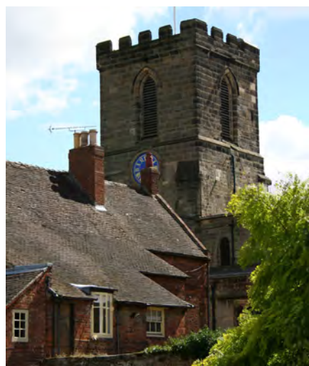
Church from Church Street
