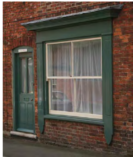
Right and above - 10 Market Place and 20 Potter Street - small "side street" shopfronts of the mid 19th century incorporating similar details; narrow pilasters, truncated at the base, a simple cornice and frieze rail and windows with glazing bars. The example at 20 Potter Street still retains its giant sash window.
