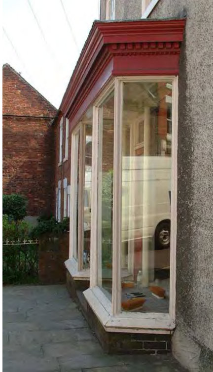
Left - refined projecting shopfront with intricate cornice, dentilled moulding and plate glass windows (25 Market Place).
