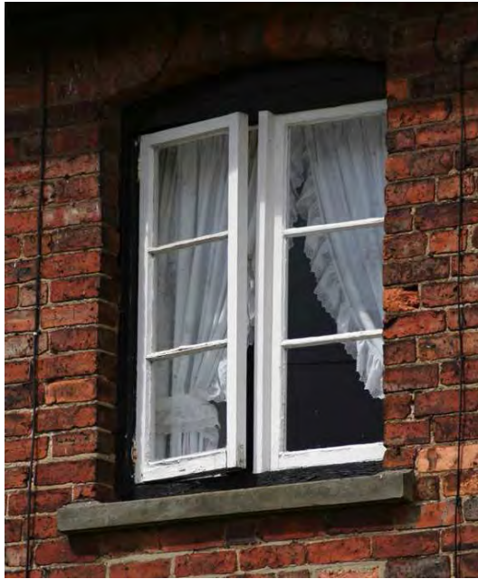
Above - side-hinged timber casements recessed within chamfered frames at Creamery Cottage.
