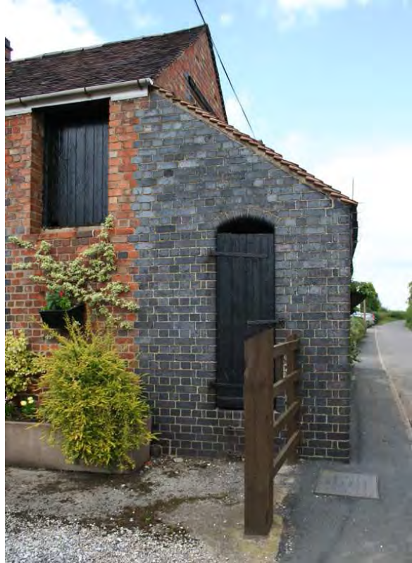
Above right - blue bricks with rounded moulded bricks adopted for the corners, where there was greatest potential for wear, at The Creamery.
