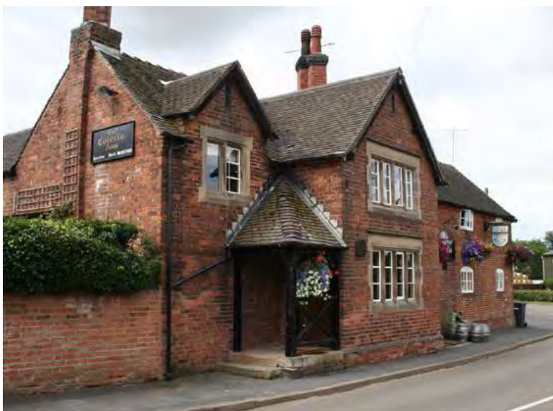
The Colville Arms - picturesque Victorian Gothic extension with stone mullioned windows
