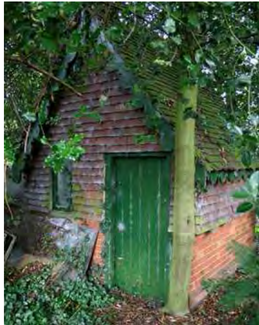
Below - decorative scrolled bargeboards and tile-hung walls at the late 19th century well-house at Lullington Hall.
