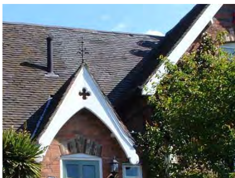
Pitched roofs - verges emphasised with shaped timber bargeboards and finials (above).
