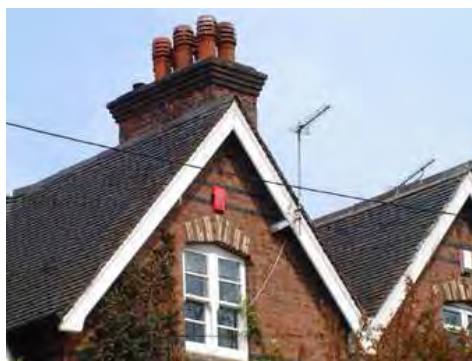
Pitched roofs - verges emphasised with shaped timber bargeboards and finials (above).
