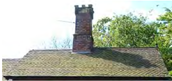
Raised coped brick gable (left) and decorative clay tiles (below) incorporating bands of plain and beaver tail tiles
