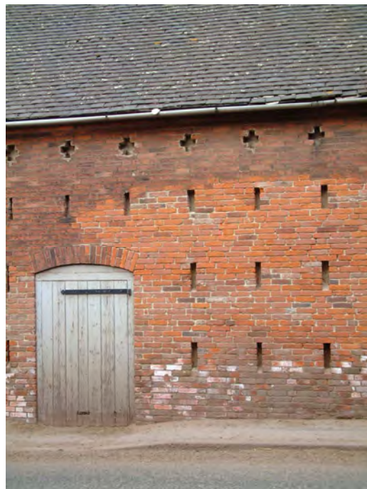
Flight holes for dovecote (left) and ventilation holes in barn (right) at Trent Farm
