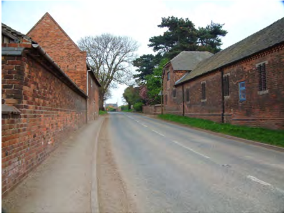
View along Repton Road between the outbuildings of Grange and Trent Farms
