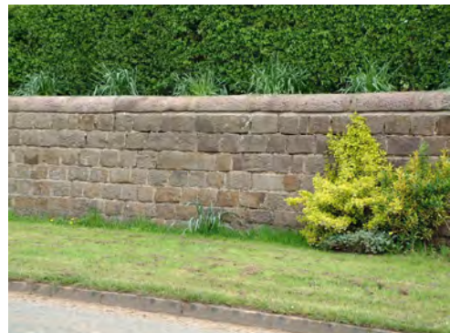
Early boundary walls were constructed from rubble sandstone, as in the example at Trent Lane (above).
