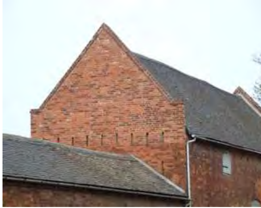
Raised coped brick gable (left) and decorative clay tiles (below) incorporating bands of plain and beaver tail tiles
