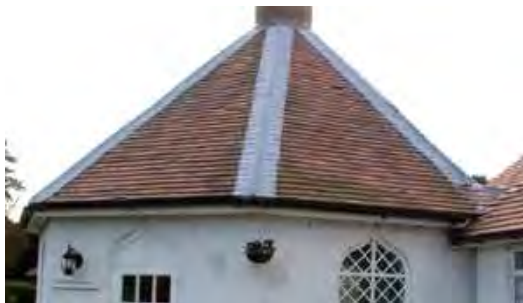
Hipped roofs - Above - hipped red clay tiled roof with lead flashings
