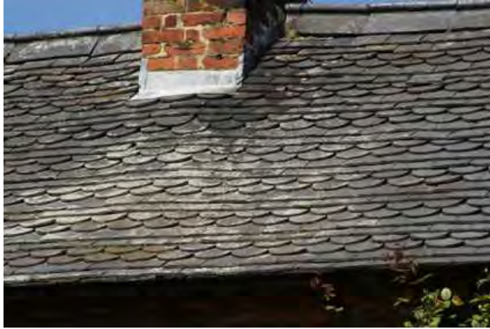
Above - Staffordshire blue clay tiles with alternating bands of fish-scale tiles at Eaton's Cottage. 19th century picturesque estate cottages often incorporated patterned tiled roofs.
