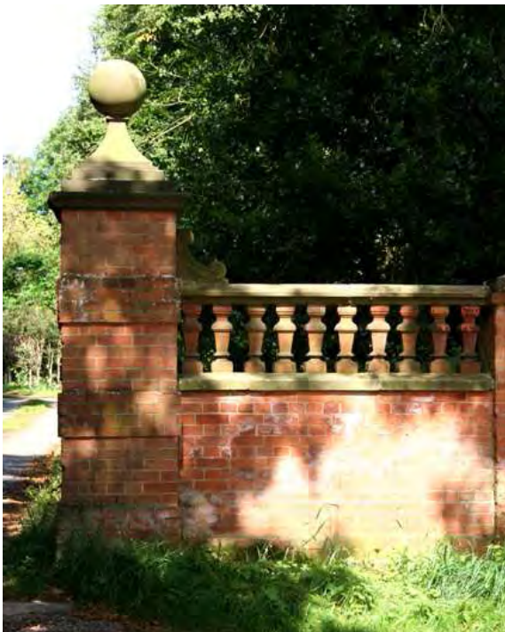
Below - 20th century brick gatepier and terracotta balusters with stone cappings and stone ball finial at Trusley Manor.
