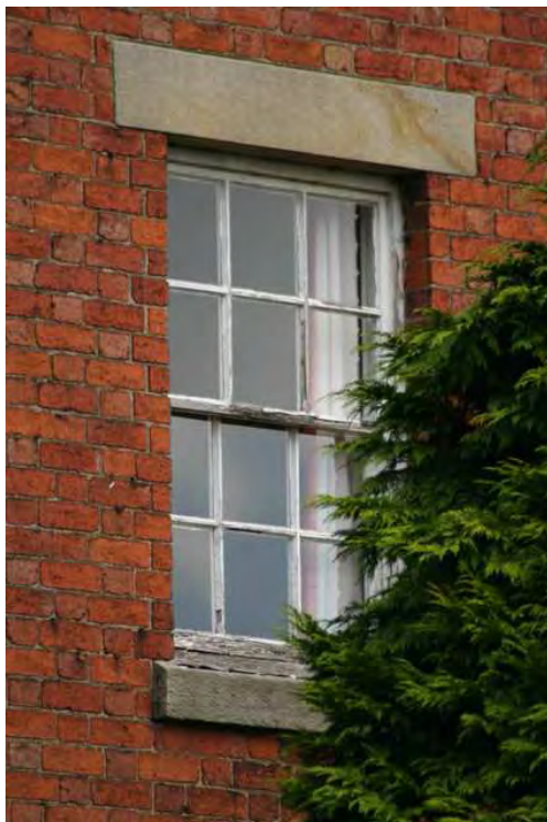
Left - Home Farm. "6 over 6" vertically sliding sash window, introduced in the 19th century, in conjunction with a stone lintel. Most of the buildings with stone lintels also have stone cills.
