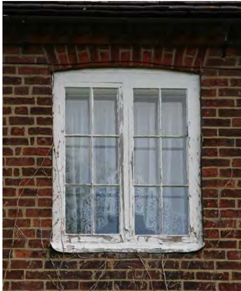
Above and right - side-hinged, small-paned timber casements at estate buildings.
