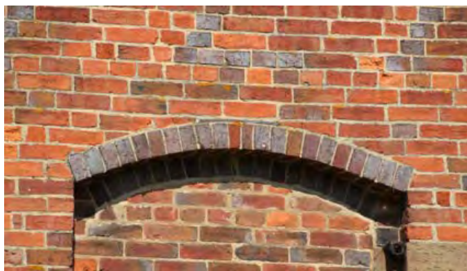
Blue “flared” (or burnt) bricks were used decoratively for their contrasting effect, such as this segmental arch lintel at Ivy Close Farm
