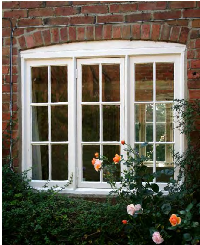
Above and right - side-hinged, small-paned timber casements at estate buildings.
