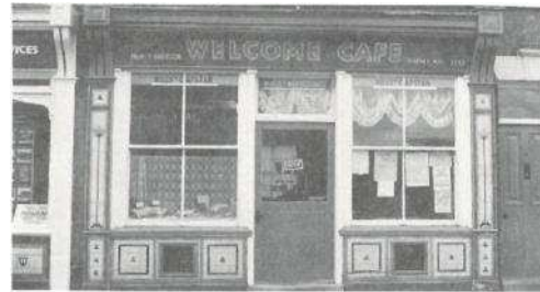
Late 19th century shop front with glazed tiling at Melbourne.
