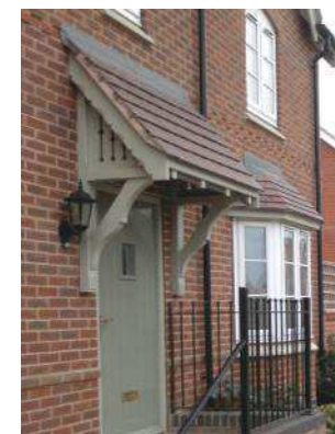
Castleton Park, Church Gresley: Timber door canopy
