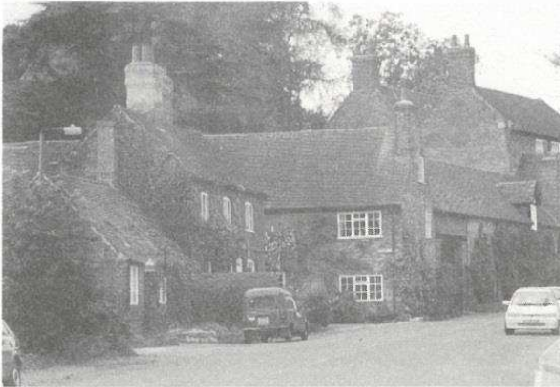
A typical grouping of traditional buildings in Melbourne. The building in the centre of the picture has unfortunately lost its original window
