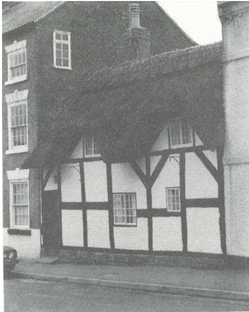
Potter Street, Melbourne. 16th century timber frame.
