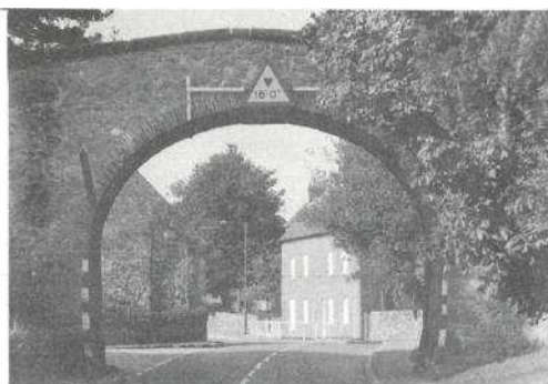
Ticknall arch (1794) which once carried a tramway is listed Grade H.
