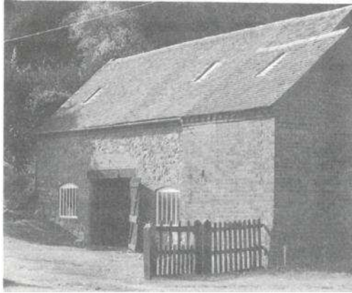
Unlisted agricultural building in Ticknall.
