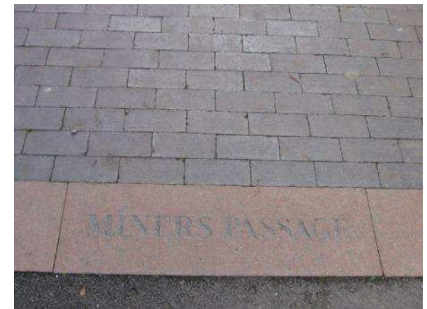
Staffordshire blue clay bricks and granite threshold strip with historic reference: Swadlincote town centre
