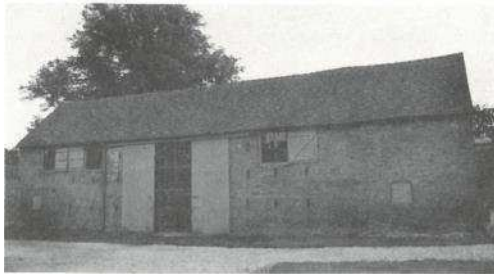
Former threshing barn, now a restaurant at Calke Abbey. Notice the 'breathers' on either side of the large doorway.
