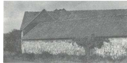
Agricultural buildings in Ticknall. Walls and roofs uninterrupted by openings.
