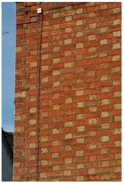
Above - 19th century Flemish bond brickwork, with buff coloured header bricks (6 Weston Road).
