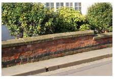
Left - at Rectory Mews moulded red and buff-coloured bricks have been incorporated into the boundary walls to create recessed panels and decorative copings, now badly eroded.
