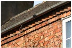
Above left and right - a sawtooth brick eaves, at 10-14 Weston Road (above left) and 22 The Green (above right).
