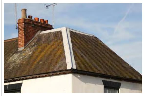
Above - hipped roof of Staffordshire blue clay tiles with hips and ridge incorporating lead flashings dressed over lead rolls (No. 1 Derby Road).
