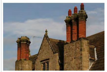
Left - red brick chimney stacks, set diagonally, with moulded stone cappings (The Hall). These chimneys were rebuilt in their original 17th century form, when the Hall was restored c1910. They are unique in the village.
