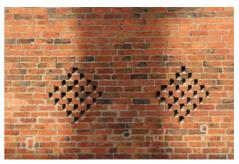
Barns needed ventilation and the diamond pattern ventilation holes adopted at Chantry Barn (above) and at Jawbone Lane (top left) were decorative as well as functional. The long, narrow slits (below) at The Hall were a simple, practical alternative.
