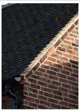
Verge finished with pair of exposed rafters, supported on wall plate and purlin ends, 12 Main Street (above left). Corbelled verges at 78 Main Street (above right).
