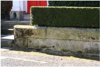
During the 19th century several frontages of the middle-sized houses were given a dwarf wall, in ashlar, with a chamfered coping, surmounted by a set of ornate iron railings. Both examples at Cofton House (above) and Chantry House (left) have lost their original railings.
