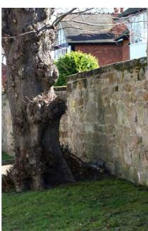
Left and far left - tall, mortared rubble gritstone walls fronting Main Street incorporate either triangular, chamfered or flat copings.
