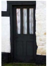
Left - panelled door with pair of flush bottom panels incorporating bead mouldings and three glazed panels separated by muntins (54 Main St).
