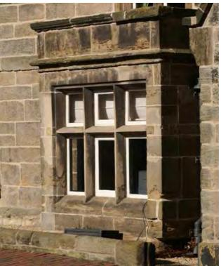
Above - bay window at Chantry House, a 19th century addition, incorporating chamfered mullions and transom, plain casements and parapet with moulded cornice.
