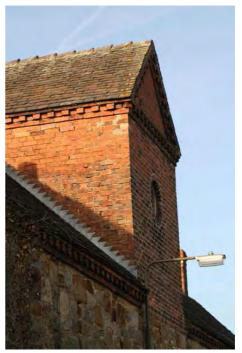
Above centre - raised brick band with "dentilled" bricks, and stone quoins, at 32 Trent Lane. Above - 18th century raised horizontal brick band (the stableblock to The Hall).
