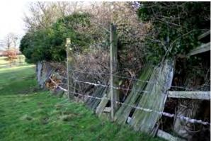
The northern fenced boundary to Kings Newton Hall grounds has partially collapsed and is in poor condition (pictured above right). It incorporates concrete stanchions, timber posts and rails and timber cladding, all repaired in barbed wire. The unkempt appearance detracts from the rest of the park and garden.
