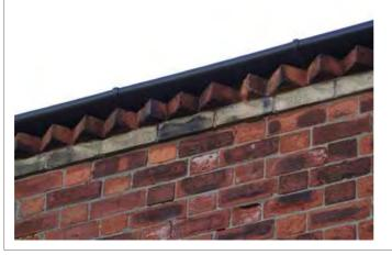
There are several types of decorative brick eaves within the village. Some incorporate brick corbelled out in a "dentilled" or "sawtooth" pattern
