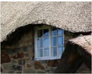
Left - along Main Street there are many examples where small gables with overhanging eaves and fascia boards were added, when the buildings were re-roofed around the turn of the 20th century. The tiled roofs replaced thatch. The only example of a thatched roof is at Manor Oak Cottage (above). The eyebrow dormer within the thatch has much softer lines than the tiled gables.
