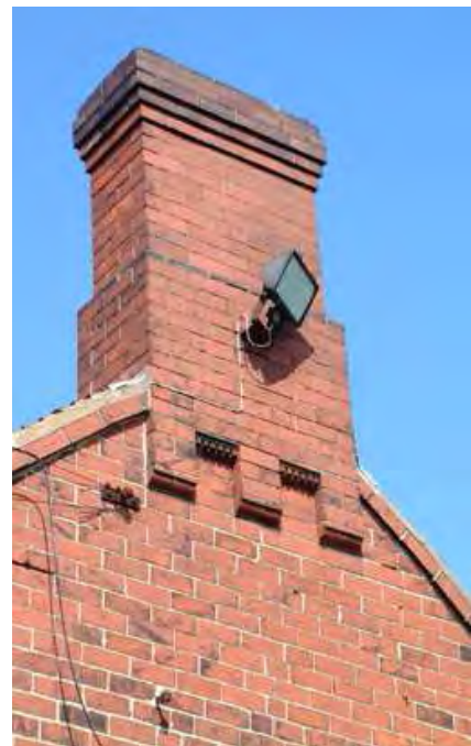
Corbelled brick stacks (right and right above)
