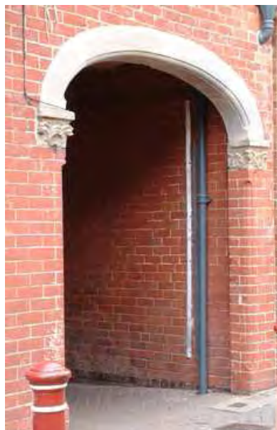
Left - three-centred stone arches, with brick piers and decorative capitals, span cart entrances
