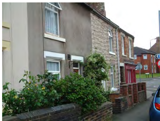
Artificial stone cladding and render over original brick
