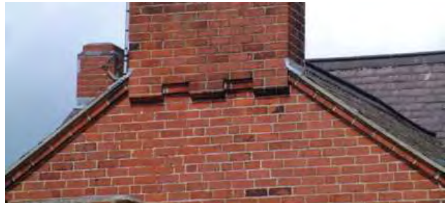
Corbelled brick stacks (right and right above)
