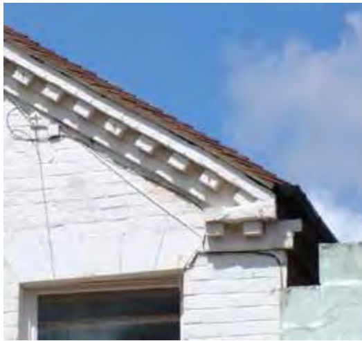
A raised brick band on the gable end of brick houses follows the verge, to provide a drip moulding (above left) and corbelled in several bands (above right)
