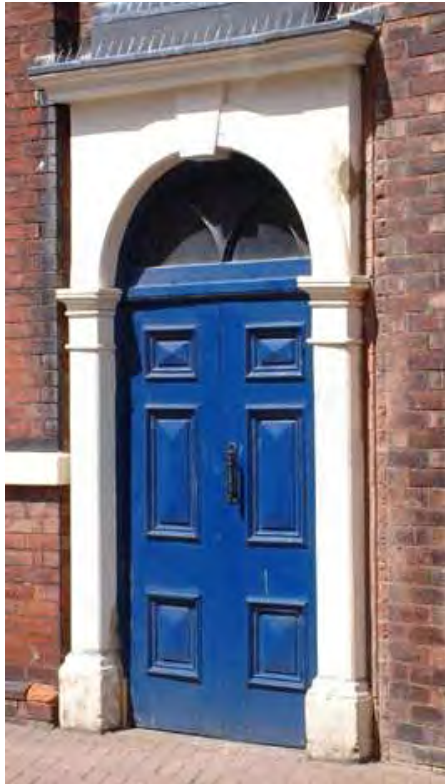
Above - pair of three-panel chapel doors, designed to reflect the proportions of Georgian six-panel doors. The panels are “raised and fielded” with bolection mouldings. The classical style doorcase is high in order to accommodate the semi-circular fanlight.
