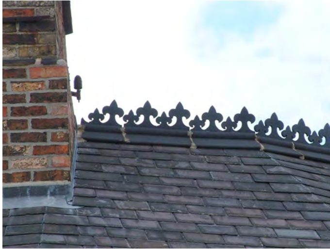
Left - decorative clay ridge tiles in blue and red clay incorporating cresting with fleur-de-lys, trefoil and roundel patterns.
