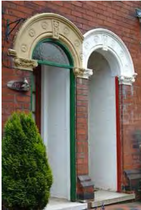
Above - painted terracotta, arched lintels to porches at Church Street
