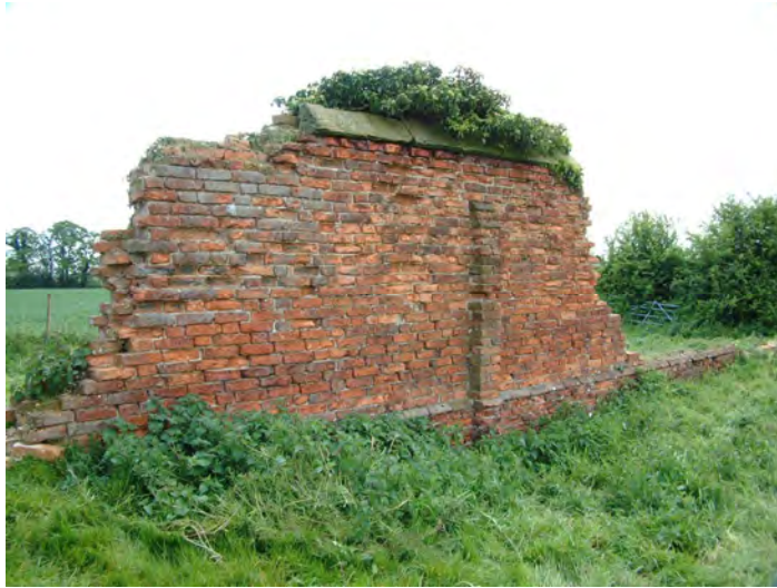
Brick boundary walls (left). These walls, built from long, thin bricks, with an ashlar coping, are fragments of the probable early 17th century kennels and kitchen garden at the former Swarkestone Old Hall.
