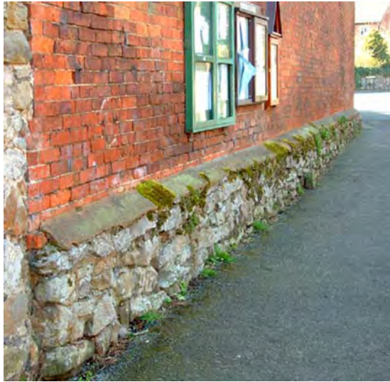
Right - rubblestone plinth, roughly coursed and dressed, with chamfered stone weathering and quoins at 40 Main Street
