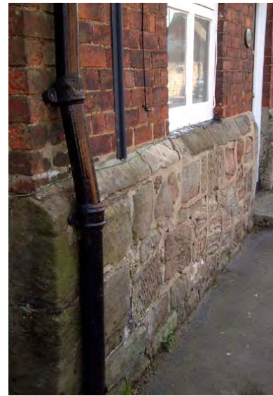
Right - rubblestone plinth, roughly coursed and dressed, with chamfered stone weathering and quoins at 40 Main Street
