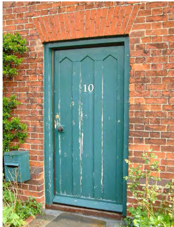
Below left - five-panel Victorian door, the bottom two panels have “scratch” mouldings, whilst the upper panels have “chamfer-stop” mouldings and “raised and fielded” panels. Slender pilastered timber doorcase with mouldings. Below right - gothic style boarded door at 10 Church Lane, with pointed arched top rail, one of only a handful surviving that were adopted by the estate.
