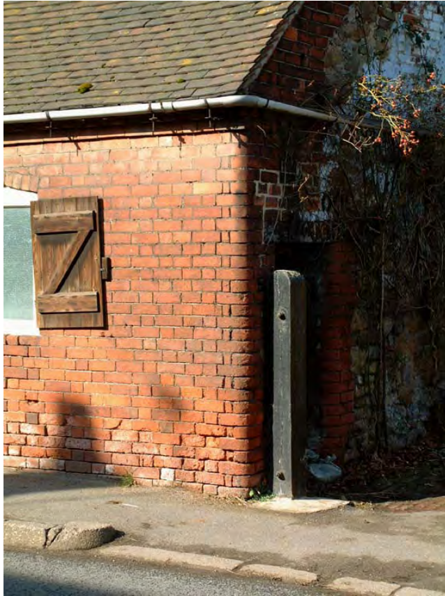
Above and left - a number of buildings and features, such as chimney stacks, were built by the estate with rounded, moulded bricks. These were handmade in special moulds.
