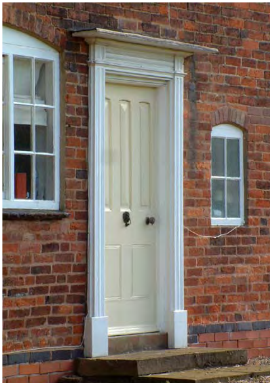
Below left - five-panel Victorian door, the bottom two panels have “scratch” mouldings, whilst the upper panels have “chamfer-stop” mouldings and “raised and fielded” panels. Slender pilastered timber doorcase with mouldings. Below right - gothic style boarded door at 10 Church Lane, with pointed arched top rail, one of only a handful surviving that were adopted by the estate.
