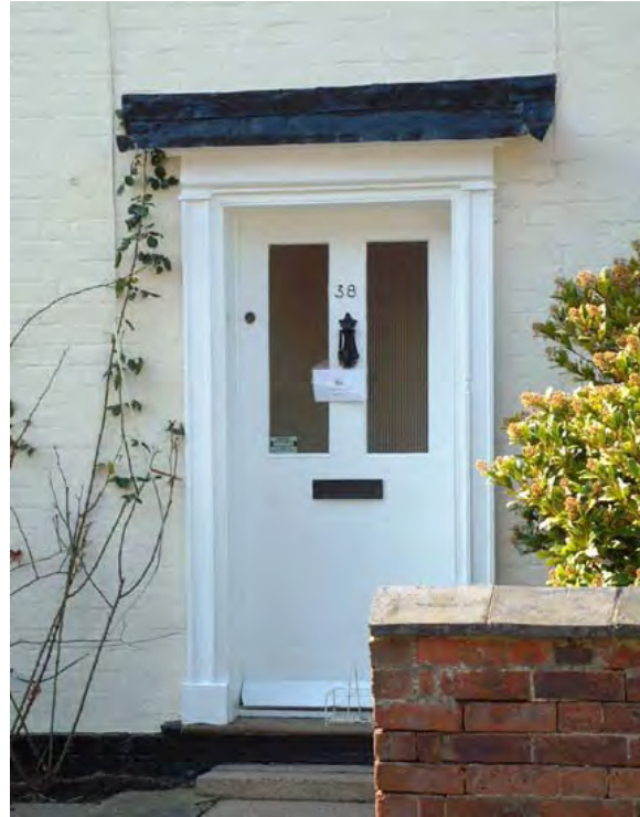
Above left - porch; a simple ornamental timber trellis with lead canopy at 35 Chapel Street. Above right - four-panel door at 38 High Street, incorporating simple “scratch” mouldings and simple doorcase with cornice.
