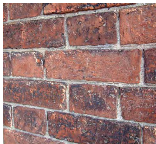
Right - "penny-struck pointing". The fresh lime mortar joints are incised with a penny, rolled in the surface to create a crisp appearance.
