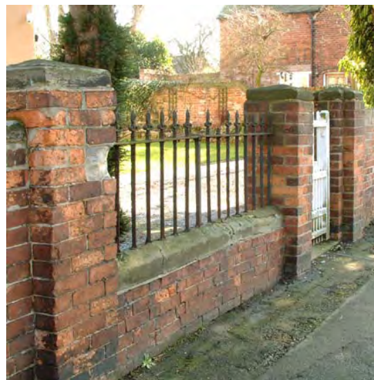
Right - in some instances wrought iron railings were combined with cast iron finials, which could be ordered by the local blacksmith from a catalogue. Here fleur-de-lys finials are combined
