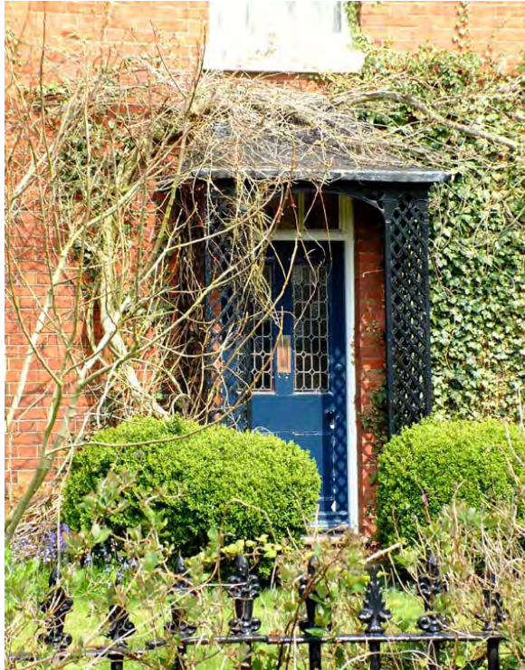
Above left - porch; a simple ornamental timber trellis with lead canopy at 35 Chapel Street. Above right - four-panel door at 38 High Street, incorporating simple “scratch” mouldings and simple doorcase with cornice.
