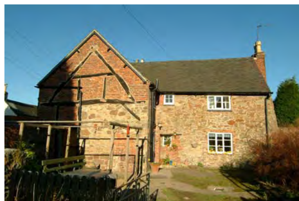
Fragment of timber frame exposed in the gable of Springfield House Farm
