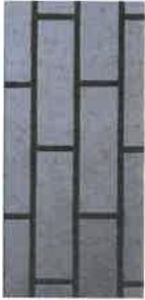
Staffordshire blue clay bricks making up curved planters
