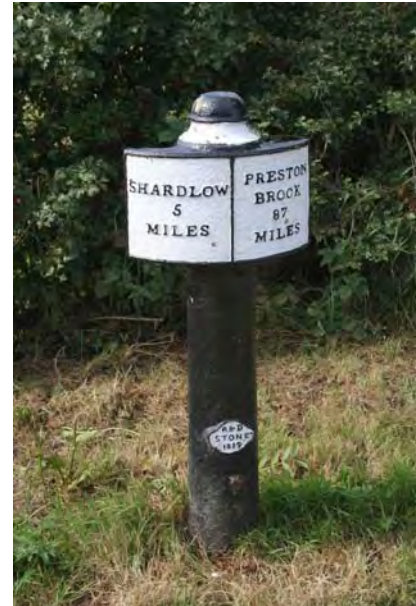
Right - Cast iron half-bobbin milepost (1819 original) with quatrefoil plaque at base, produced by Rangeley and Dixon of Stone.
