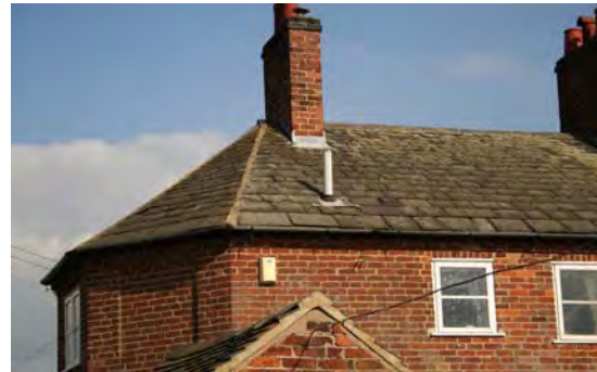
Above right - hipped graduated Westmoreland slate roof with mitred hips at Swarkestone Stop.
