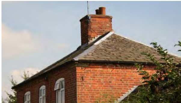
Above left - hipped graduated Westmoreland slate roof with lead flashings (probably covering failed mitred hips) at Lock House, Swarkestone.
