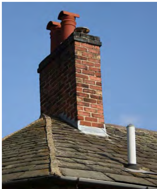
Left - brick stack with rounded moulded corners (Stenson Lock - Harpur Crewe estate). Blue brick oversailing courses (above) at Swarkestone Stop.
