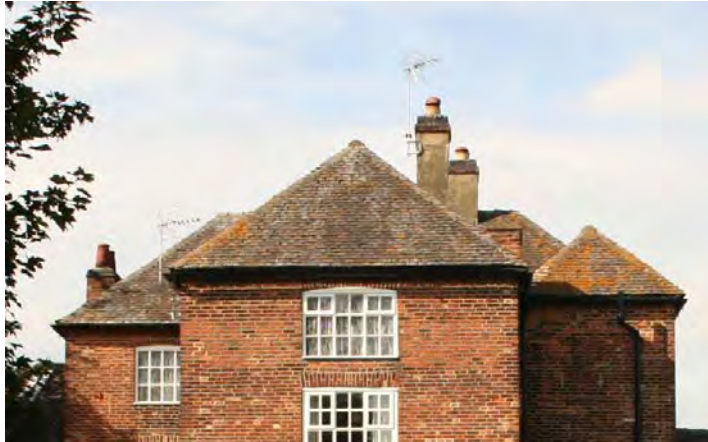
Left - hipped tiled roofs, with bonnet tiles cloaking the hips, at Weston Grange. Hand-made red clay tiles were used in this area before the arrival of the canal, but the exact origins of this house are slightly obscure.
