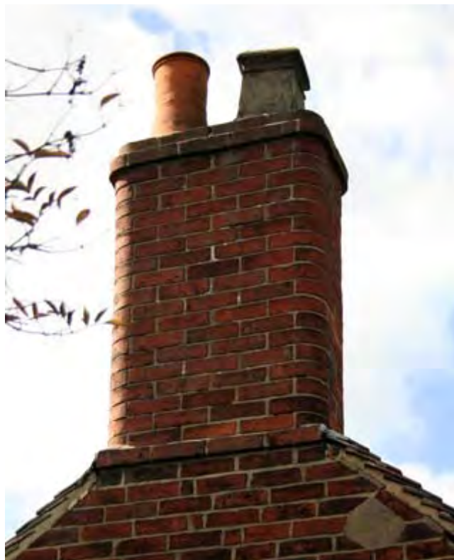
Left - brick stack with rounded moulded corners (Stenson Lock - Harpur Crewe estate). Blue brick oversailing courses (above) at Swarkestone Stop.
