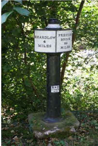
Left - Cast iron half-bobbin milepost (1819 original) with square plaque at base, produced by Rangeley and Dixon of Stone.
