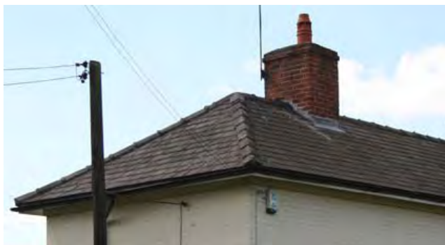
Above - hipped Welsh slate roof with overhanging eaves and tiled hips (Lock House, Stenson Lock).
