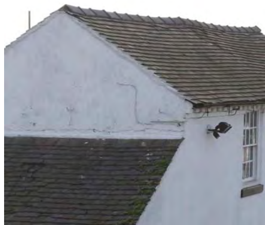
Above - hipped Welsh slate roof with overhanging eaves and tiled hips (Lock House, Stenson Lock).
