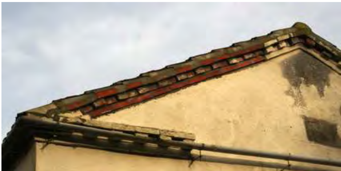
Below - gable-fronted elevation of the former chapel on Chapel Lane. The corbelled and dentilled brick verge continues part way along the front elevation.
