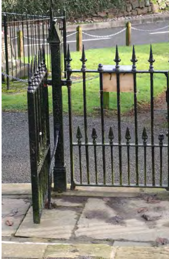
Above left and top right - cast iron railings and gates with spear-headed finials at St. James Church. Above right - hooped steel railings with finials at Hamilton House, Chapel Lane.
