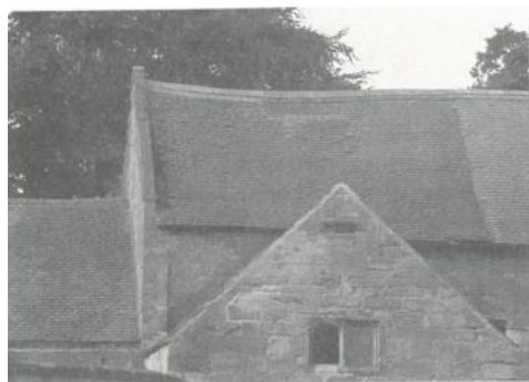
Melbourne Tythe Barn. A mixture of brick, stone, machine made and hand made plain clay tiles.
