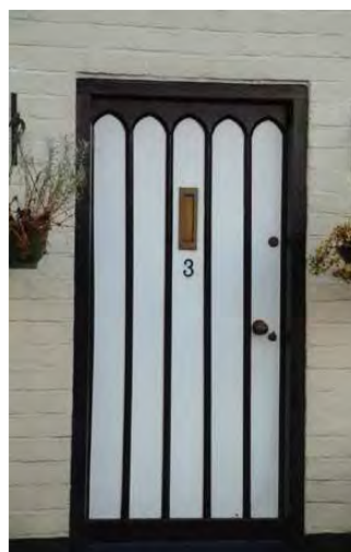
The Gothic Revival introduced a range of doors - nine-panel within a pointed arch (left), plank door with applied fillets and pointed Gothic arches (above centre) and boarded within a pointed arch (above right).
