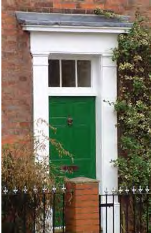
Six-panel door with simple “bead” mouldings (above), incorporating fanlight and Georgian style classical doorcase with cornice, frieze rail and plain pilasters.
