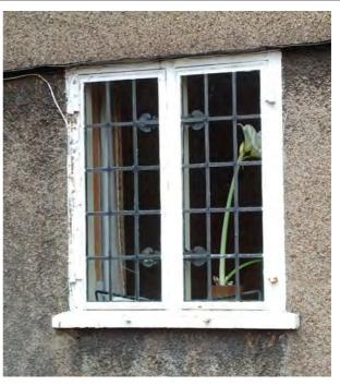
The first windows were made with glass "quarries" (square or diamond-shaped pieces of glass), separated by lead "cames". The lozenge shape evolved as a result of the process of making crown glass. By the 18<sup>th</sup> century, glass quarries were usually rectangular in shape (as at The Old Priory - left).
