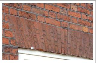
In the 18th century, where wealth permitted in the finer houses, "hand-rubbed" bricks or "gauged" bricks were used. The result was a precise, thinly-jointed, wedge-shaped lintel. Originally, the brickwork joints (including false joints) were picked out in a fine white lime mortar or "putty", which in most cases has weathered away (left and above). The example at 50 High Street (below) is an early 20th century copy.
