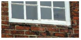
Above - where there was no cill, as with many of the smaller cottages and the less important elevations of the town houses, the window joinery was positioned close to the face of the wall. In the example above handmade bricks were moulded to create a weathering.
