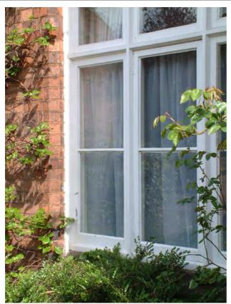
Windows with hinged opening lights are known as casements. Early opening lights were generally of wrought or cast iron and were often designed to carry leaded lights. By the late 18th century timber opening lights with glazing bars were becoming more common and sometimes replaced the earlier metal ones.
