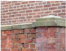
The earliest walls within the village are built from local stone, the best examples being the large blocks of stone used for the Priory precinct walls, which have wedge-shaped stone copings (right), but there are instances where rubble sandstone survives, usually on the side passages, sometimes freestanding & sometimes used for the footings of a later 18<sup>th</sup> or 19<sup>th</sup> century wall (right).
