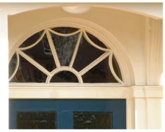
Fanlights were used to light a hallway, which was often otherwise unlit, and became common when house plans changed to incorporate a central hallway with a staircase in the Georgian period. Until then, doors generally opened onto a small lobby or directly into a room and there was no need for the additional light source.
