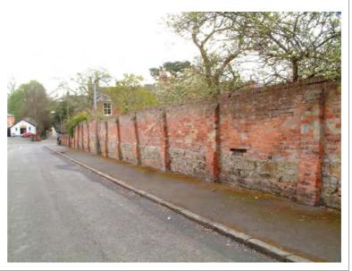
Most of the boundary walls serving domestic properties within Repton are built from red brick, with a sparing use of headers to form the bonding pattern. The example on the right is a late 19th century wall to The Priory, using English Garden Wall bond brickwork and red clay copings on an earlier wall.
