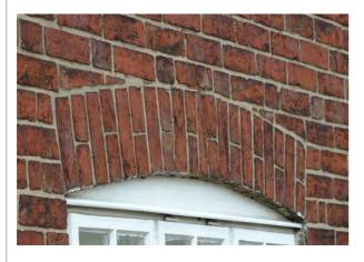
Simpler segmental arched lintels are more common, formed by a course of "stretcher and header" bricks (14 Brook End - left). For the cheapest type of construction, the arches were half the height, using a single row of header bricks.
