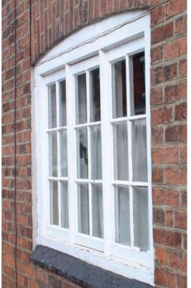
The cast-iron casements at 100-104 High Street (left) were designed in a gothic style to mimic the leaded-light quarries of traditional leaded-light windows, but in the 19<sup>th</sup> century, by using cast-iron, they could be made more cheaply by mass production. They differ in appearance from their leaded predecessors, because the glazing bars in a cast iron window were usually painted
