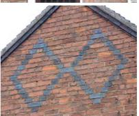
Polychromatic brickwork using blue bricks (above), and occasionally buff, was used in the second half of the 19th century in Repton. At 8-10 Well Lane (above right) a simplistic diaper pattern on the gable end with hood moulds in blue brick, echoing Tudor brickwork, distinguishes the building above the ordinary.
