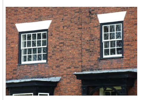
Brook Farm (above), with exposed sash boxes and wedge lintels. There are hints that the lintels are formed with render over original segmental arches, and that the sashes are a later alteration, replacing original casement windows.
