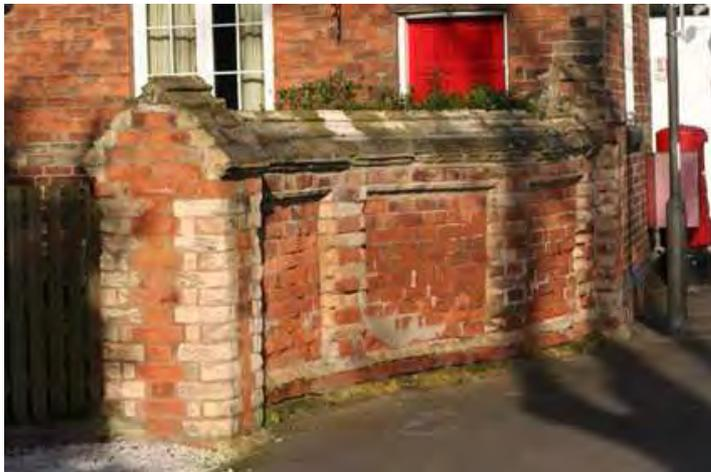
Left - at Rectory Mews moulded red and buff-coloured bricks have been incorporated into the boundary walls to create recessed panels and decorative copings, now badly eroded.
