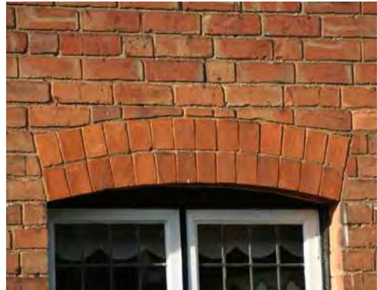
There was often no cill, relying on the weathering properties of the brickwork. Window joinery was positioned close to the face of the wall. Lead cills may be added for improved weathering if desired. (below - 2 Weston Road).
