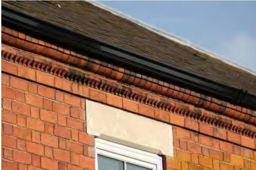
Left - moulded terracotta eaves at 4 The Woodlands. This type of eaves typically has a cast iron ogee gutter. This sits on top of the projecting eaves, avoiding the need for brackets. The shaped gutter is therefore an integral part of the architecture of the building.
