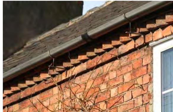
Above left and right - a sawtooth brick eaves, at 10-14 Weston Road (above left) and 22 The Green (above right).
