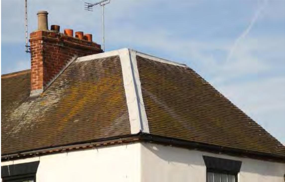
Above - hipped roof of Staffordshire blue clay tiles with hips and ridge incorporating lead flashings dressed over lead rolls (No. 1 Derby Road).
