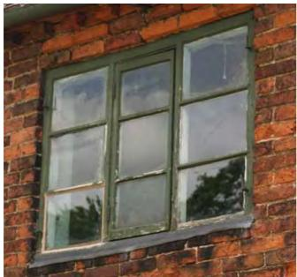
In many instances there is neither a lintel nor a cill, as in the outbuilding at the Old Hall (left). Instead the brickwork above the window is supported on the window frame. The cill has been simply protected here, at a later date, with a lead flashing.
