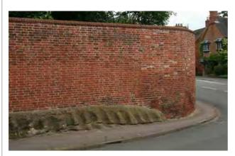
Above - The old wall on the corner of Church Street and Main Street was built on top of the bedrock. The wall at the entrance to Newlands House (right) was part built in rubble sandstone. In both cases moulded red brick copings were used. They were ideally suited to following the undulating wall head (detail below).
