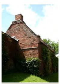
Stepped brick parapet to roof at Grade II listed former Smithy at the Old Stableyard
