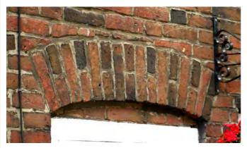
In association with casement windows, the most common pattern of lintel is the segmental brick arch. This was often used for economy. The example at The Almshouses (left) incorporates header and stretcher bricks, many of the headers have been fired at a higher temperature and so appear almost blue. The brick infill between the arch and the window, set back, is a typical early detail.
