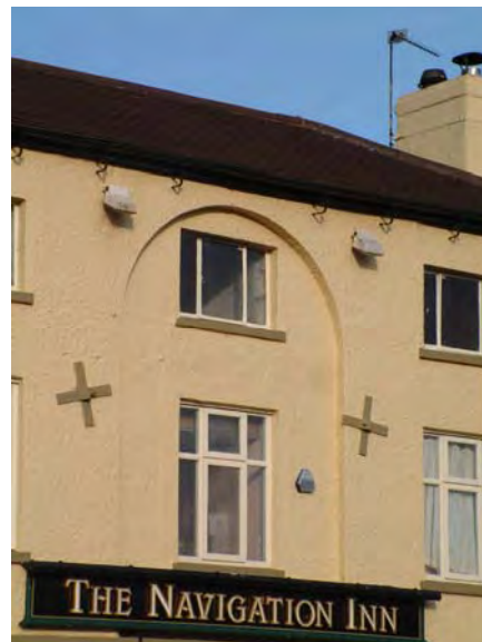
Loss of sash windows and textured render
