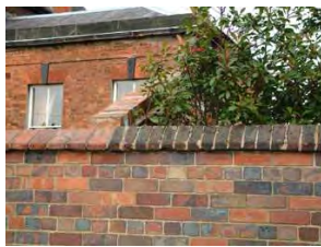
Half-round and triangular coping details (above).
