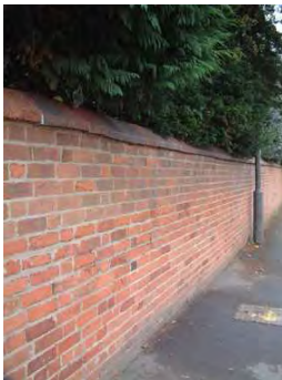
Half-round and triangular coping details (above).
