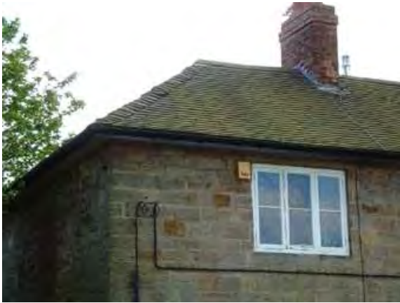
Above left - hipped roof in Staffordshire blue clay tiles with bonnet tiles to the hips
