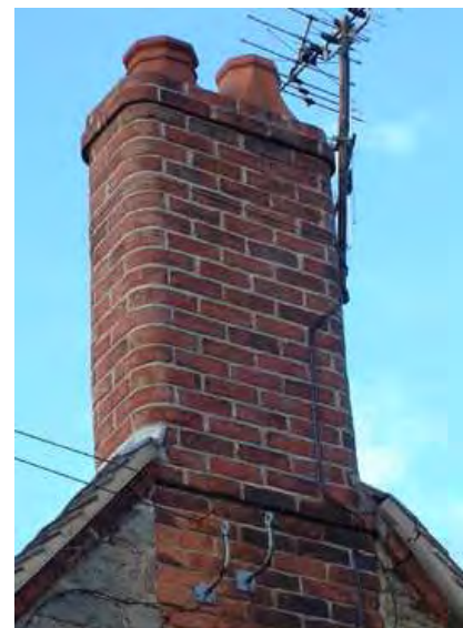
Rounded moulded bricks - used in conjunction with brick chimney stack (right) and corner of agricultural building (above)
