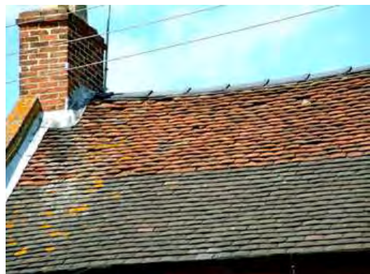
Below right - roof incorporating mixture of old handmade plain red clay tiles and Staffordshire blue clay tiles
