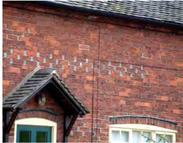
Above and right - the pattern of ventilation holes within brickwork is distinctive. They are survivals from the original use of buildings as hay barns. Most of these slots have been blocked up with slate or blue bricks when the buildings were converted from agricultural uses into dwellings.
