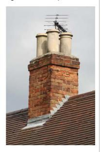
Blue bricks were occasionally used when a stronger brick was required, especially in architect-designed Victorian buildings. Blue bricks were fired at higher temperatures and were more durable. They were ideal for oversailing courses. Blue bricks were mainly introduced in the second half of the 19th century, principally on practical grounds, but on occasion they were also used decoratively. Picture, below left - chimney with moulded blue brick bands & weatherings at
