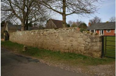
Boundary walls are commonly built from rubble gritstone, with roughly squared flat copings (left). On occasion large blocks of gritstone can be found, as at Trent House (above), which also retains its wrought iron railings, and at Water's Edge (below left).
