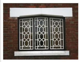
Above - side-hinged casement windows of 1864, manufactured in cast iron, at the Old Post
