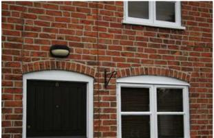
Segmental brick arches were commonly adopted in the 18th and early 19th centuries. This example at Trent House, Church Lane (left), incorporates incised stretcher bricks; each alternate brick is incised with a scratched horizontal line to receive a narrow "joint" of lime putty. The putty would have been added later to create the effect of an arch made of stretcher and header bricks. Modern repointing has removed some of the original
