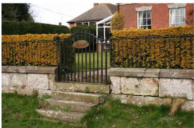
Left - decorative wrought-iron railings, with cast-iron urn finials fixed to the posts at Manor House, Church Lane. Each upright baluster is fixed into the chamfered stone coping using molten lead.
