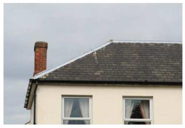
Below and bottom right - steep pitched roofs and raised coped gables. Common form of raised brick parapet at Millstone Cottage (bottom right) and Victorian Jacobean form of raised gables with moulded stone copings, at the former village school (below).
